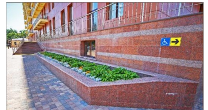
Flower beds at the central entrance new 11-storey dormitory of SSAU, decorated by specialists
