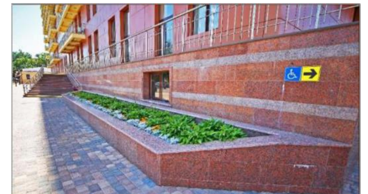
Flower beds at the central entrance new 11-storey dormitory of SSAU, decorated by specialists
